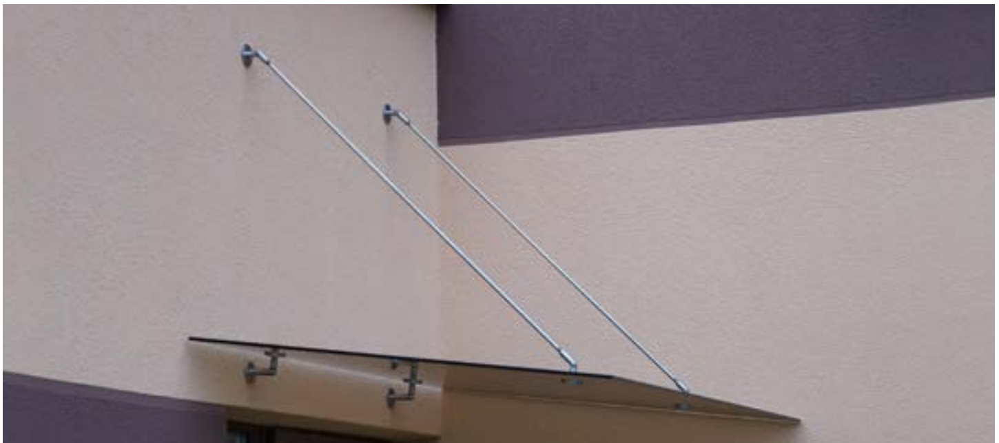
Wall To Glass Type Canopy System
